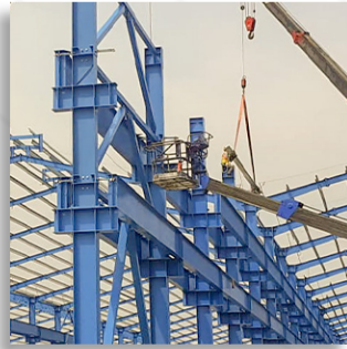
Beam Installation
