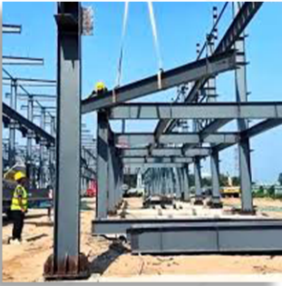
Column Erection
