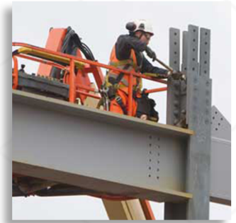
Bolt Tightening
